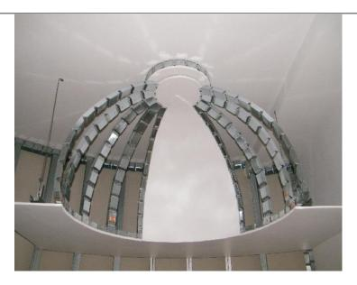
N.B.: If the dome is very big, it is necessary to place some more CONCAV Studs to strengthen the structure behind. Place them across the CONCAV already in place (double metal framework) and fix them behind the first ones with channel hangers.
