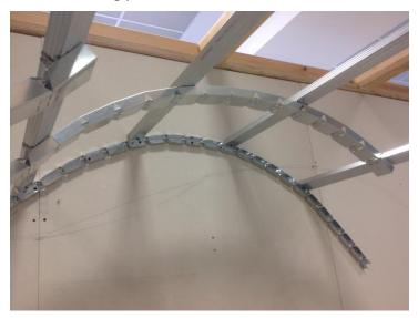
connect the Studs with a channel connector 60x27 to obtain the curvature with the desired radius
