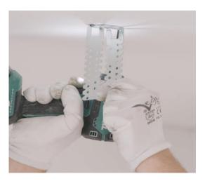
• Fix the standard studs on one side to the COBRA 30 mm fixed to the lower side of the downstand, and on the other side to the universal brackets
