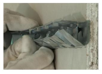
build the vault with a double metal framework: for the primary structure use C49x27 (or C60x27), for the secondary structure use the CONCAV Curving Stud and channel hangers (as for a flat ceiling)
